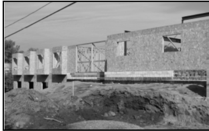
Ronald McDonald House near Sanford Health campus being constructed in October 2008.
